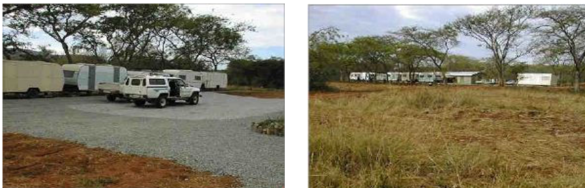
Figure 2: Examples of typical Eskom construction camps
