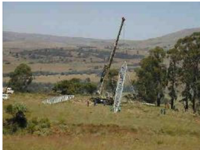
Raising the pylon
